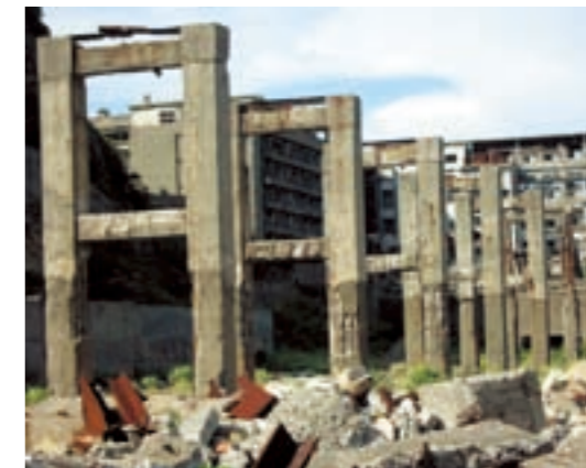
Coal Storage Conveyor Belt
