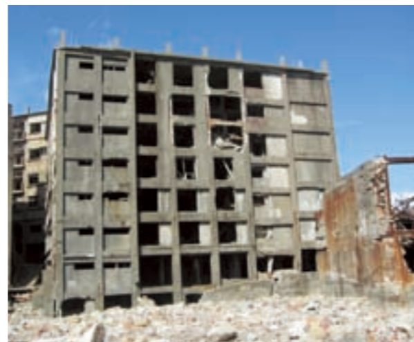
No. 30 and No. 31 Apartment Buildings
